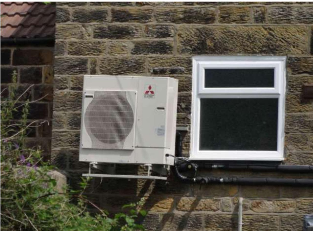
Plate 2 The heat pump adjacent to the bathroom window. All external pipes are well insulated.
