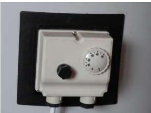
Plate 4 The water temperature controller on the hot water cylinder.
