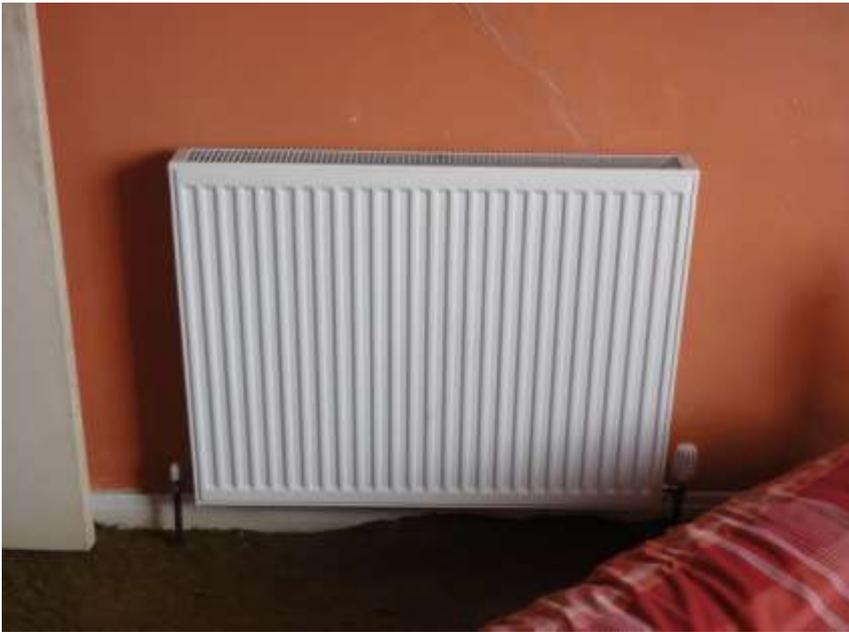
Plate 3 One of the new double convector radiators with thermostatic radiator valve.
