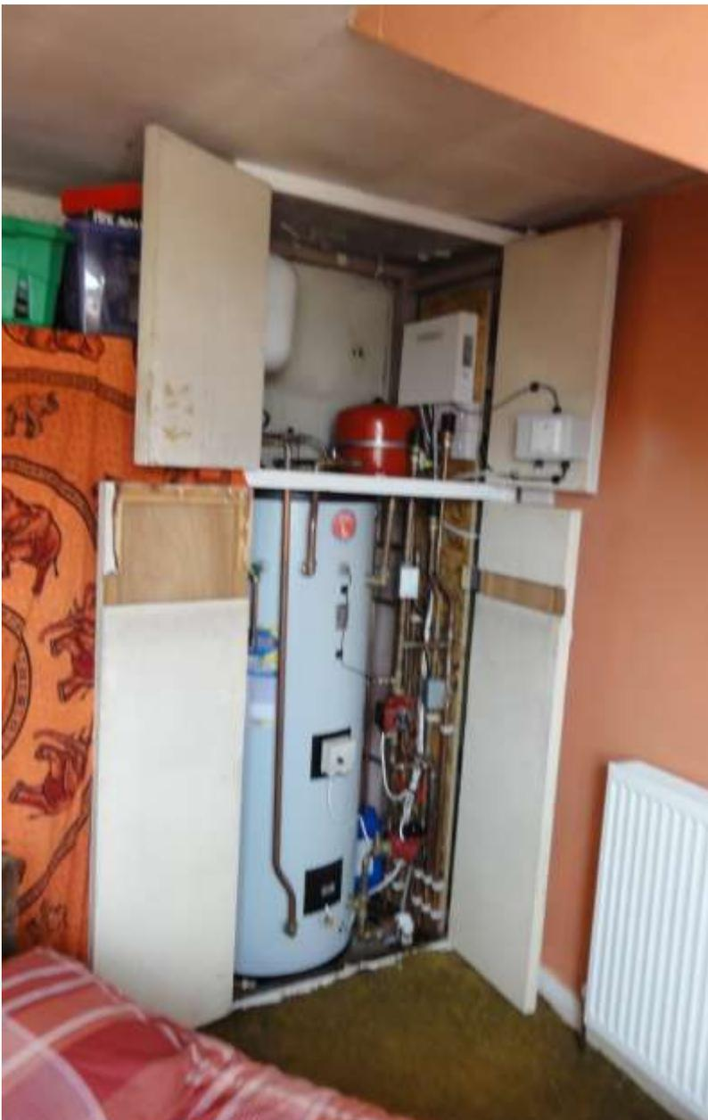
Plate 5 The hot water storage cylinder and ancillary components in the former airing cupboard.
